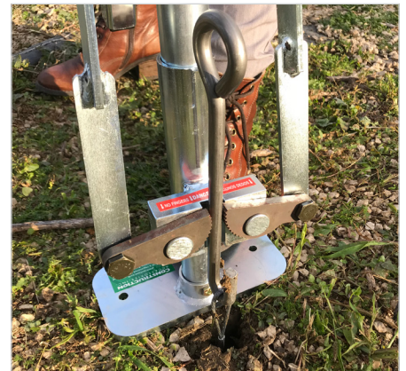
Load-locking the Anchor using the Loop Puller for Vineyard and Orchards trellising
